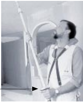
Disk added to handle—reduces grip force needed to hold and use the roller
